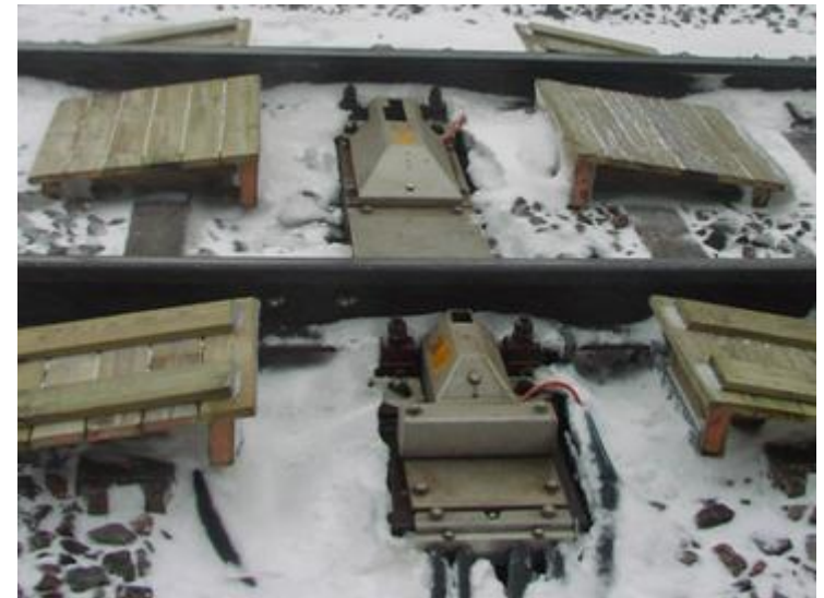
Hot Box/Hot Wheel detector
